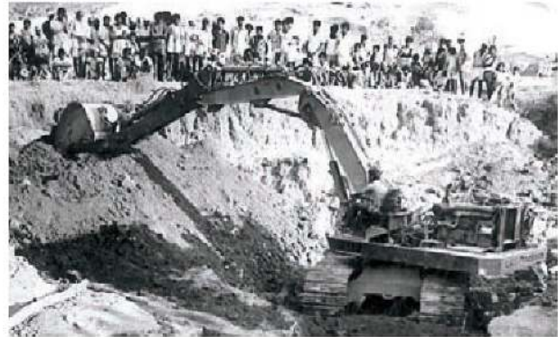
Crowds gather to eagerly watch a Hydraulic Excavator in operation
